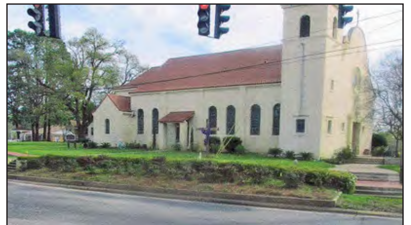
St. John's Catholic Church photographed in March 2016 from the same angle as the 1941 photograph. (Robertson Collection)
